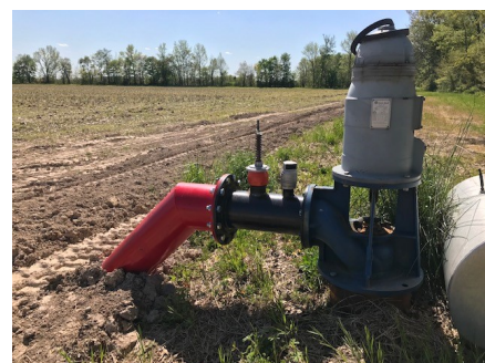
Well attached to underground pipe
