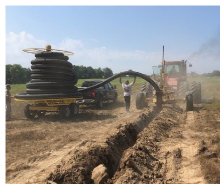
Installation of sub-irrigation pipe
